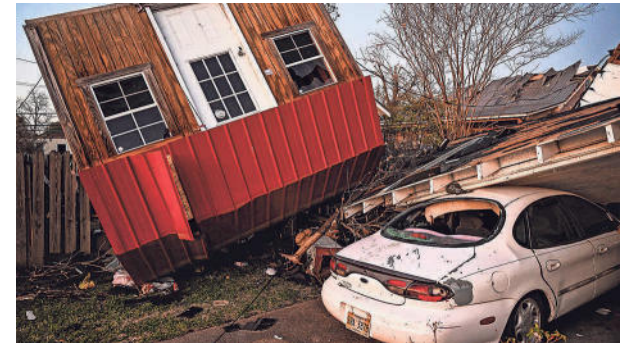
The remains of crushed houses and cars are seen in Rolling Fork, Miss., on Saturday, after a tornado hit the area. CHANDAN KHANNA/AFP VIA GETTY IMAGES
